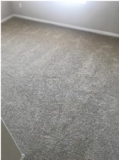
Flooring/Baseboard Taken on: 2018-09-14 17:21:00 Taken at: 33.9568345361, -117.601606291 Image
