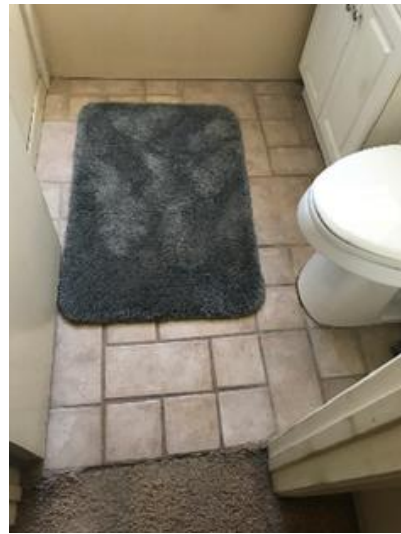
Flooring/Baseboard Taken on: 2018-07-30 10:31:10 Taken at: 33.8723454569, -117.90377682 Image
